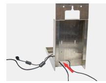
1. Feed the printer power cord and USB cable through the bottom opening.
