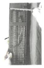
Replace front cover by sliding in the two top tabs and fastening the two mounting screws.
