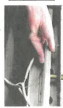
Carefully re-run the wiring through the back of the heater.
