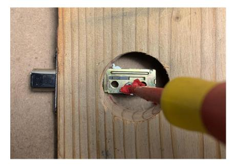
Begin by testing the deadbolt. Use a flathead screwdriver, placing it in the cross-slot on the deadbolt. Rotate the screwdriver to flip the bolt back and forth. If the bolt moves freely, skip to the next page.
