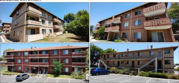
Overall condition - fair. There was a variety of conditions amongst building elements within this category. Items such as downpipes and gutters appeared to be in good condition, whilst the fascia and metal balustrades were of poor condition.
