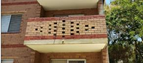
Overall condition - poor. Urgent repointing to sections of brickwork are required (notably the balustrades on upper floor levels). These areas are a safety hazard, and reinstatment of these building components in the near future is recommended.
