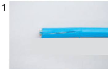
1 Expose inner vinyl sheath.
