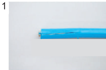
1 Expose inner vinyl sheath.
