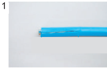
Expose inner vinyl sheath.
