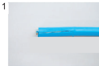
1 Expose inner vinyl sheath.
