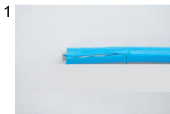
1 Expose inner vinyl sheath.
